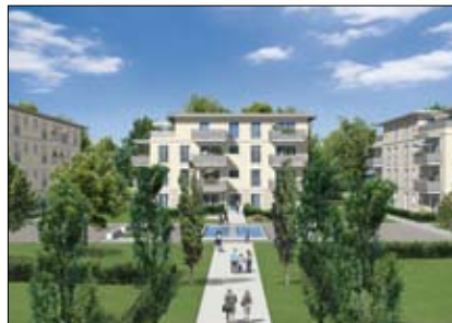
Baufeld 2 Concept Bau-Premier + SBR Arch.
